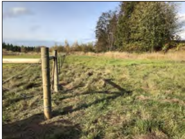
Livestock exclusion fencing recently completed. Planting will occur in early 2019.
